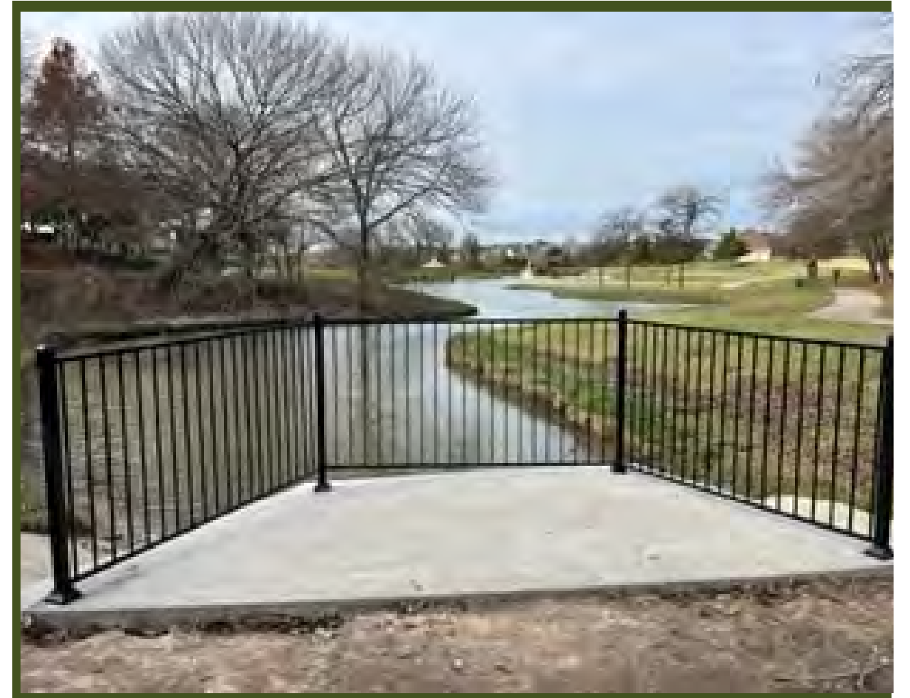
EMERALD BAY METAL FENCE INSTALL
